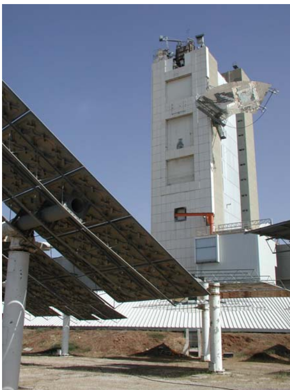
Figure 7: View from the heliostat field to the solar tower at the Weizmann Institute of Science in Rehovot/Israel. Mounted on the right side of the tower is the hyperbolic beam down mirror, which reflects the concentrated solar light coming from the heliostats into a secondary concentrator (CPC) in the white building below. The Solzinc pilot plant will be installed underneath this CPC.
